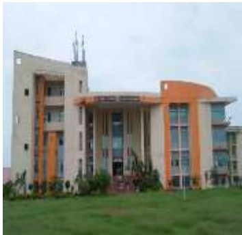
(a) Academic block (Temporary campus)
